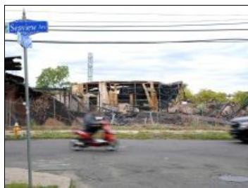
Fire hits abandoned warehouse
